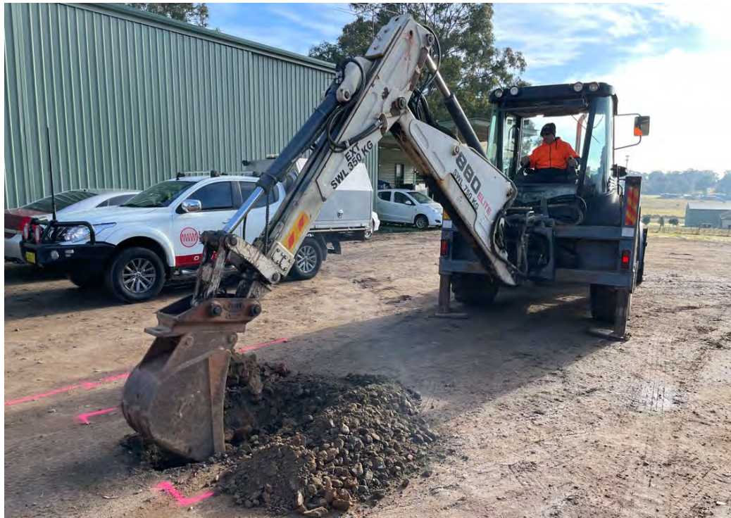
Photo 1 - Terex 880 Elite Backhoe excavating TP12_1 at Site 3 (Lot 12)
