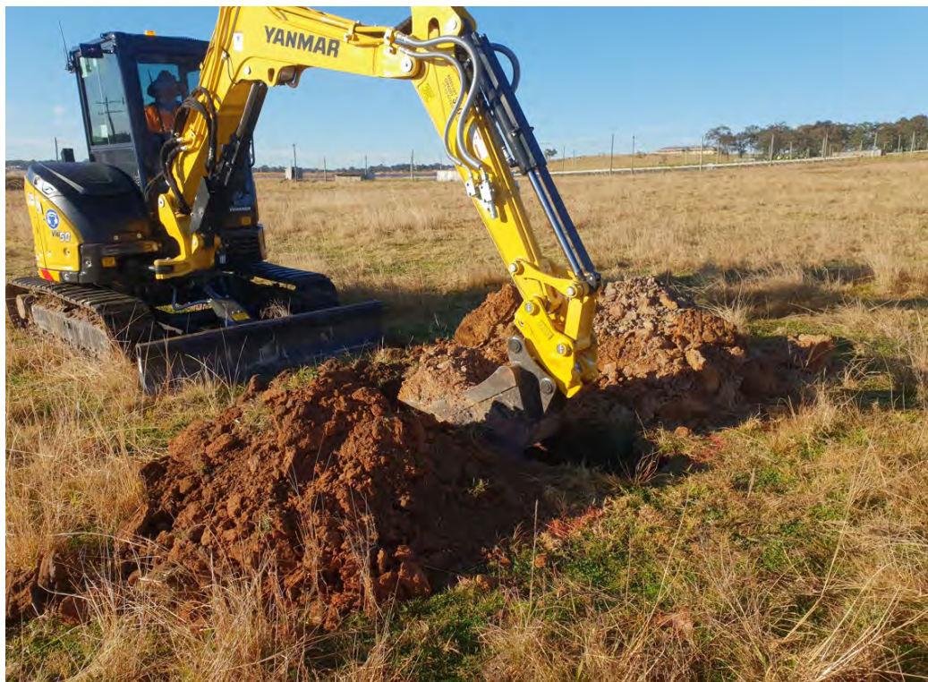
Photo 2 - Yanmar ViO50 Backhoe excavating TP11_6 at Site 1 (Lot 11)
