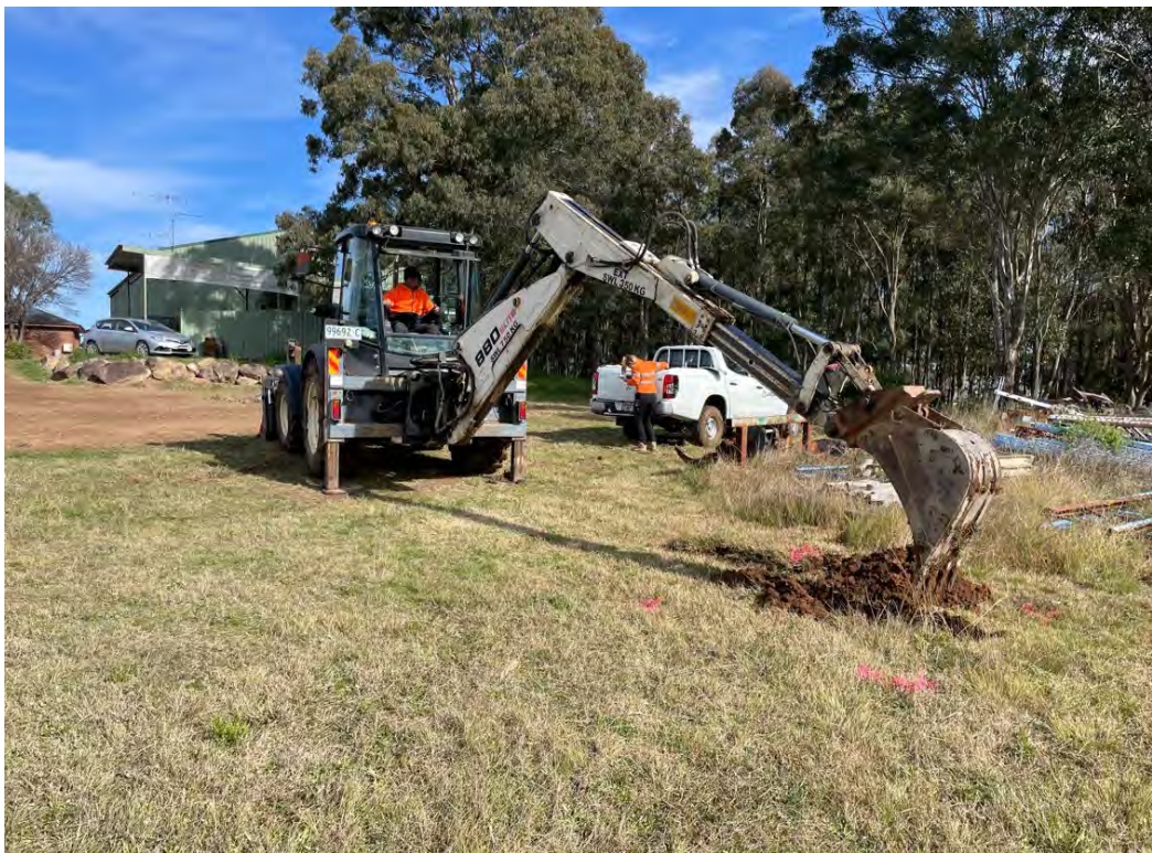
Photo 8 - Typical site conditions in Site 3 (Lot 12)
