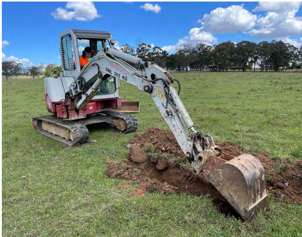
Photo 16 - Takeuchi Backhoe excavating TP13_4 at Site 9 (Lot 13)
